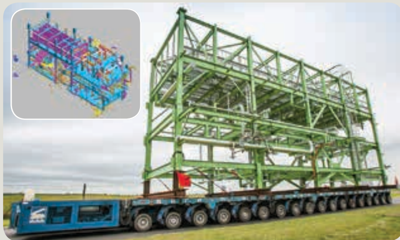
One of 26 plant modules for Sasol's CTFE plant in Secunda under construction at Hydra-Arc's Sky-Hill facility near Secunda. Inset: A 3D CAD model of Unit 296, the 158 t coal tar filtration (CTF) east filter press plant, the largest and most impressive module yet delivered.
